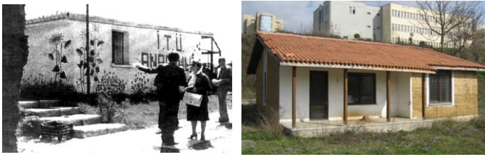
Figure 8-9. Experimental I (left) and Experimental Building II (right)
